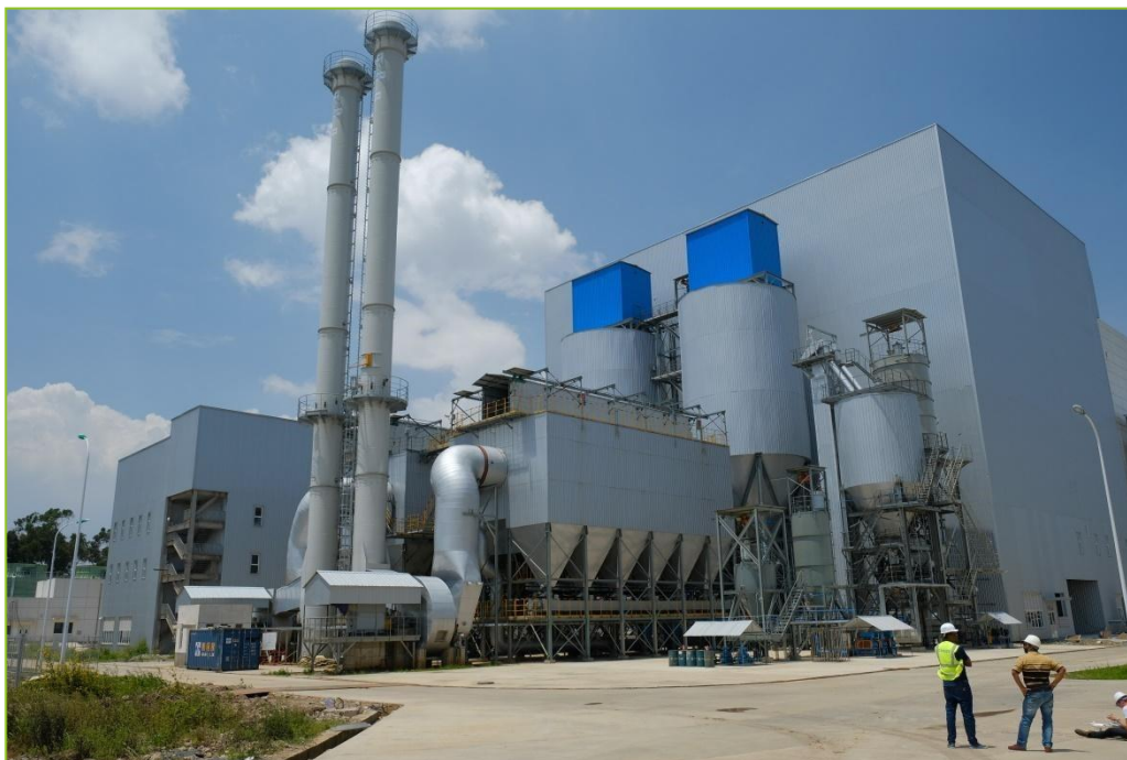
Figure 101 Reppie Waste-to-Energy facility
